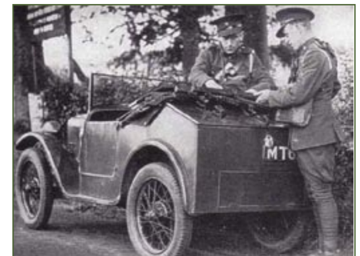
An Austin Motor Company shot showing a later car from the rear. Just visible are clips for rifles on the lid of the tail.
